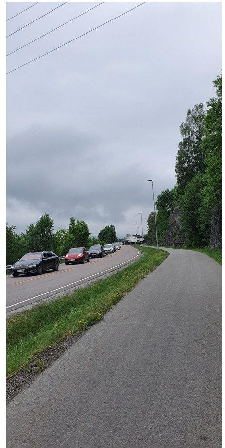
The current section of Nedre Rælingsvei Street features a physically separated pedestrian and bicycle path, enhancing the safety of road users in the pilot
