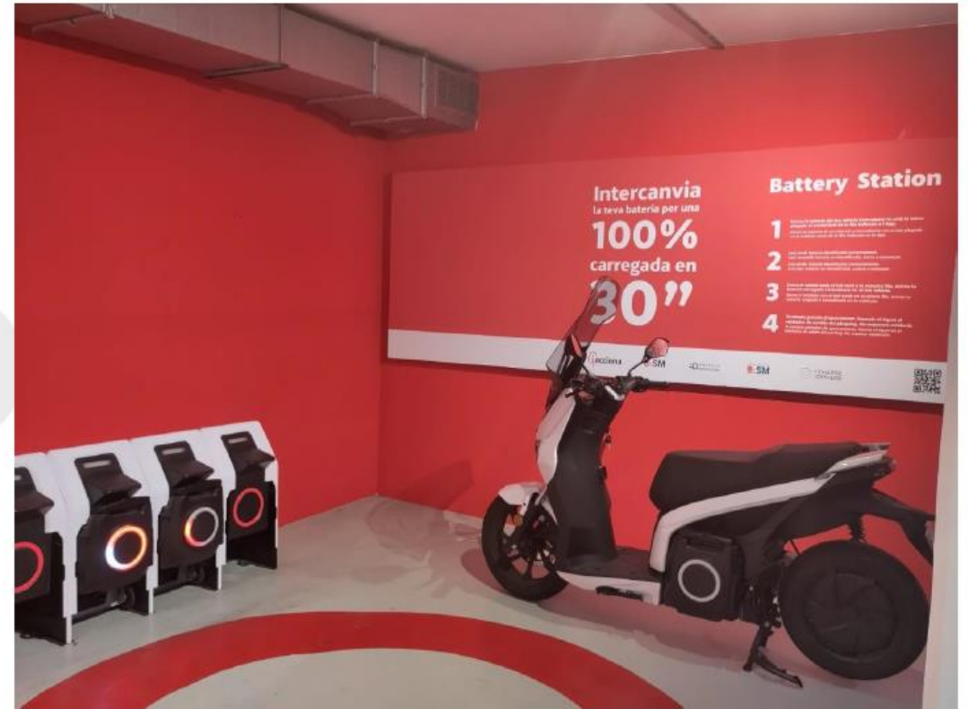
Navas Car park battery station
