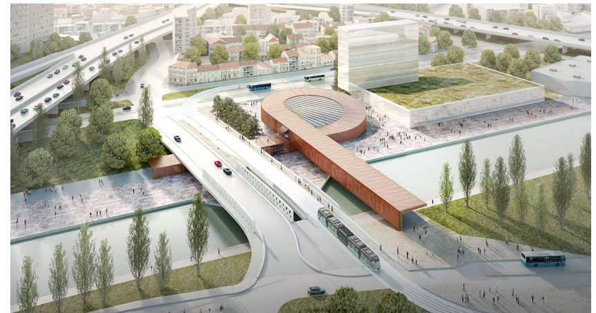
The Bondy station on the GPE network
