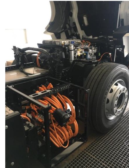
HV-power distribution unit
