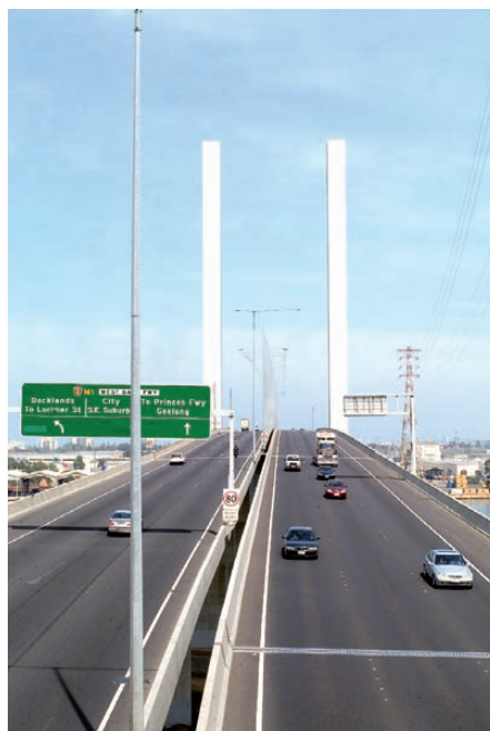
Urban Multilane Free Flow tolling in Melbourne, Australia
