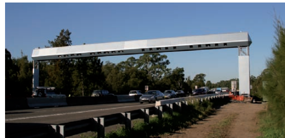
Sydney's M5 South West Motorway operates an urban MLFF system
