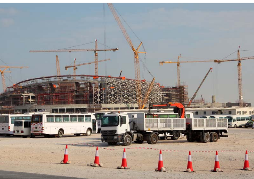
Stadium construction, Doha, Qatar
