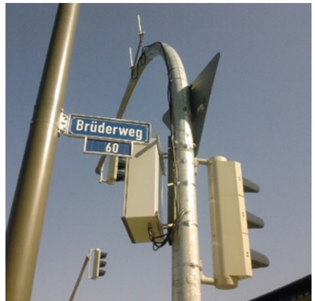
Interoperability: a vehicle unit from Spain should be able to communicate with this RSU in Germany. Source: PTV
