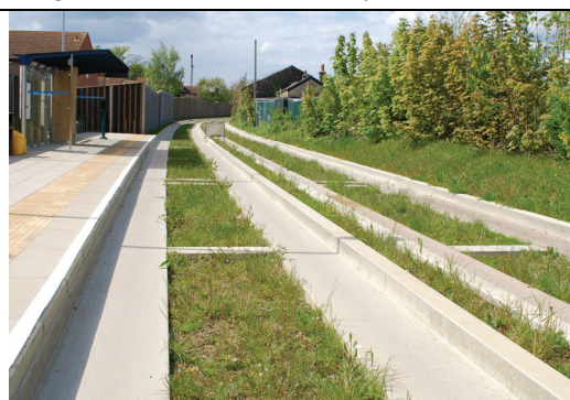
Cambridge: the guideway in concrete allows a cheap maintenance all along the 40 km, without the need for rainwater pipes
