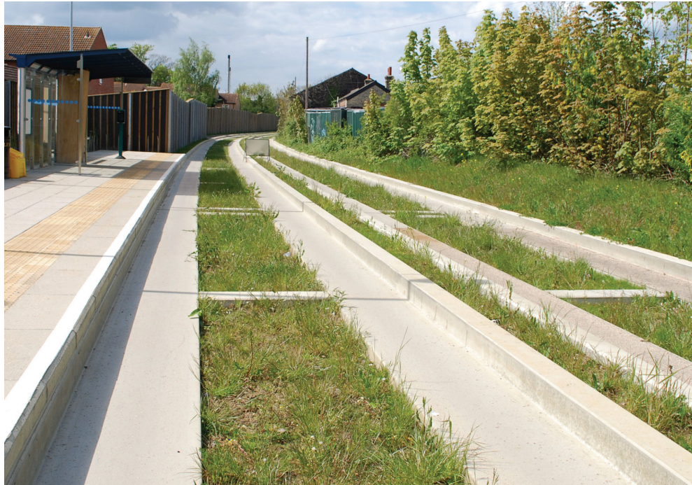
The concrete guided way along a station
