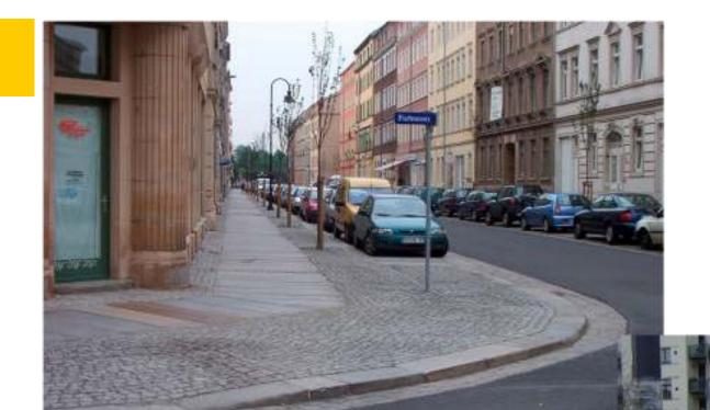
barrier-free dropped kerb with warning surface
