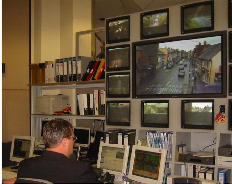
Trained members of staff are also on hand to monitor the system and put out relevant information when it is needed by travellers, transport operators and event managers. A workstation of the UTMC database is set up at Reading Football Club's Madejski Stadium, where fans can quickly be diverted between car parks as queues increase and fans arriving by public transport are guided onto dedicated buses to shuttle them between the stadium and Reading Station.
